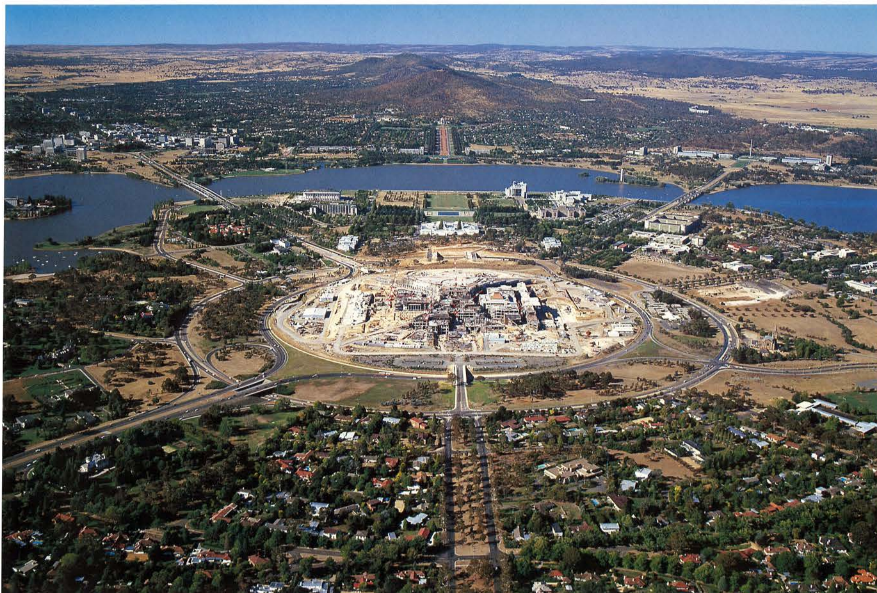
Parliament House, Canberra, under construction. Photograph 1985 by Leo Meier. WELDON TRANNIES
